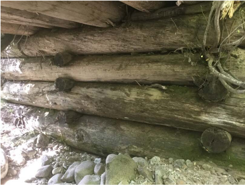
Right Bank Abutment when facing downstream
