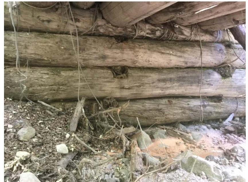
Left Bank Abutment when facing downstream
